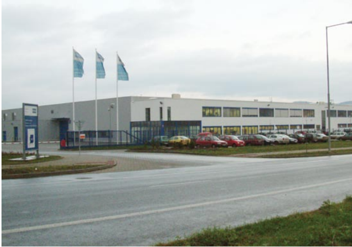
KONE, manufacturing facility in Usti nad Labem
