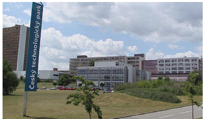
Brno Technology Park hosts the EMEA Shared Services Centre of Motorola
